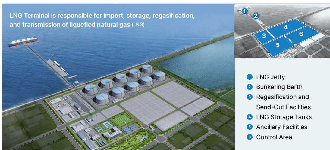
[Figure 3] Structure of LNG Terminal
